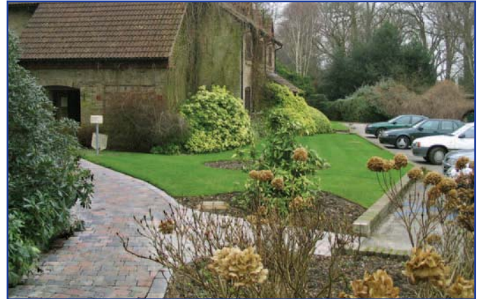
Accessible route from car park, using carefully selected 'wheelchair friendly' paving
