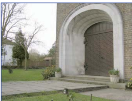
St Anselms Church before access improvement work
