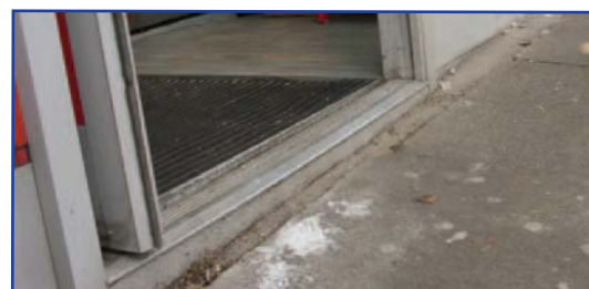
Previous stepped entrance
